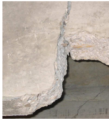
d) Rupture of the Lower Tendon
