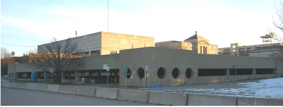
a) Side View of Parking Garage
