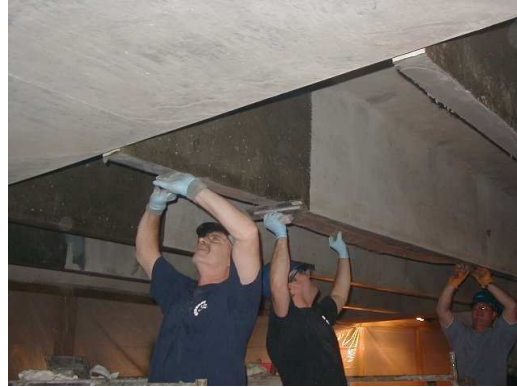
b) Application of Longitudinal Ply
