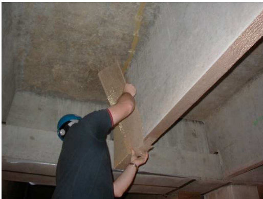
e) Application of U-Wraps
