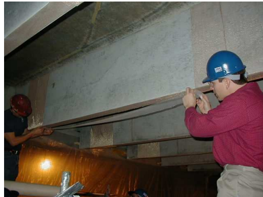
d) Application of Scrim on Longitudinal Ply
