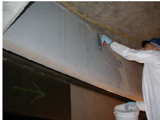
f) Application of Epoxy on U-Wrap
