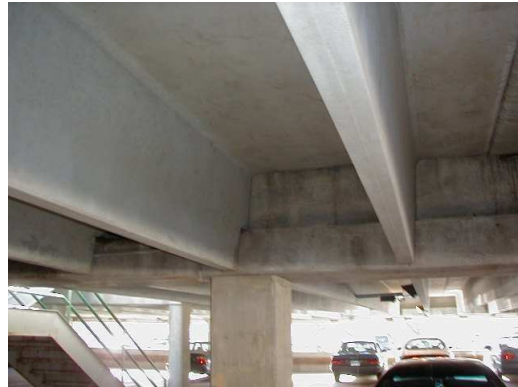
c) Bottom View of the Deck
