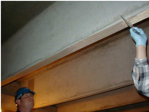
c) Squeezing Out the Resin Excess
