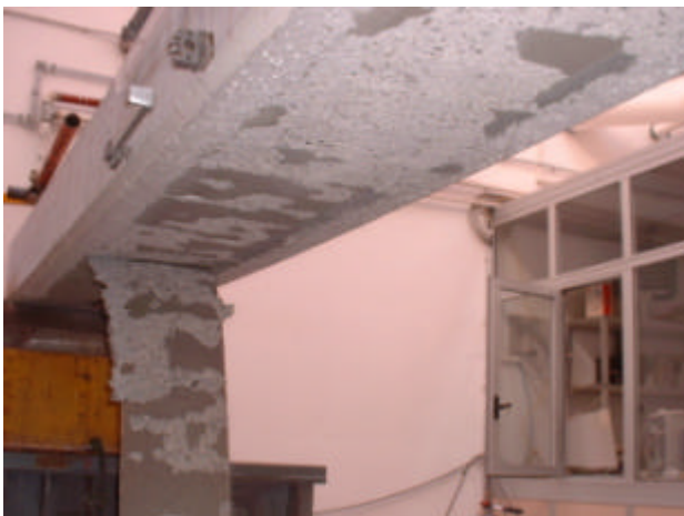
Figure 12: Bottom View of Failure of B-2 Beam
